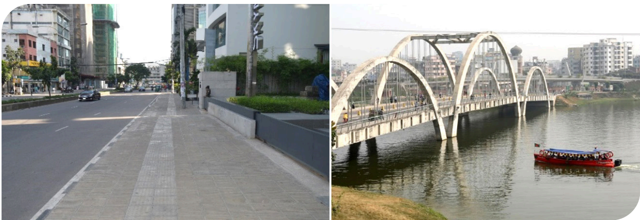
Redeveloped Footpath in Gulshan Area
